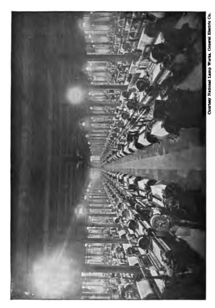
Illumination in a Weaving Room. (One 60-watt lamp for each group of four looms.)
